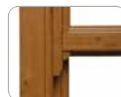
Run through sash horns
